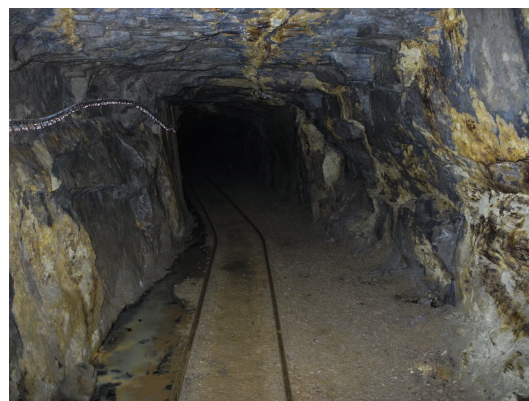
Fig. 43: Sludge and rails - Mining RoX Project
