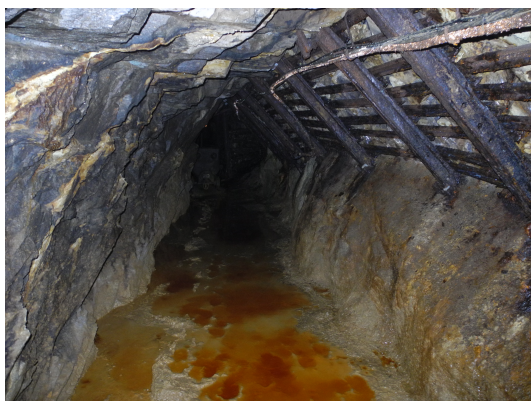
Fig. 42: Water in Mining - Mining RoX Project
